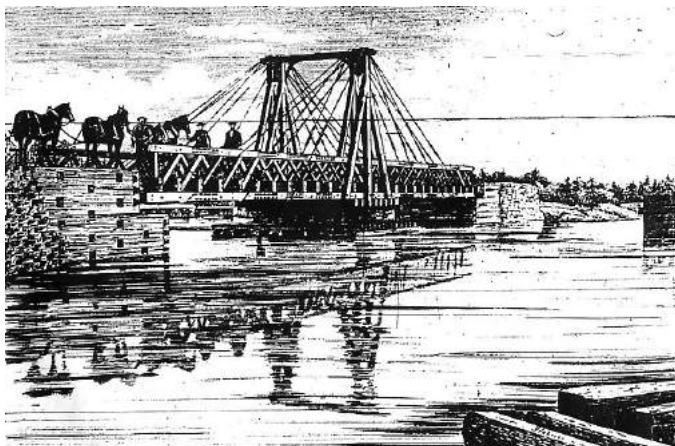
Cable-stayed railway swing bridge, Dow's Lake, Ottawa - 1871
