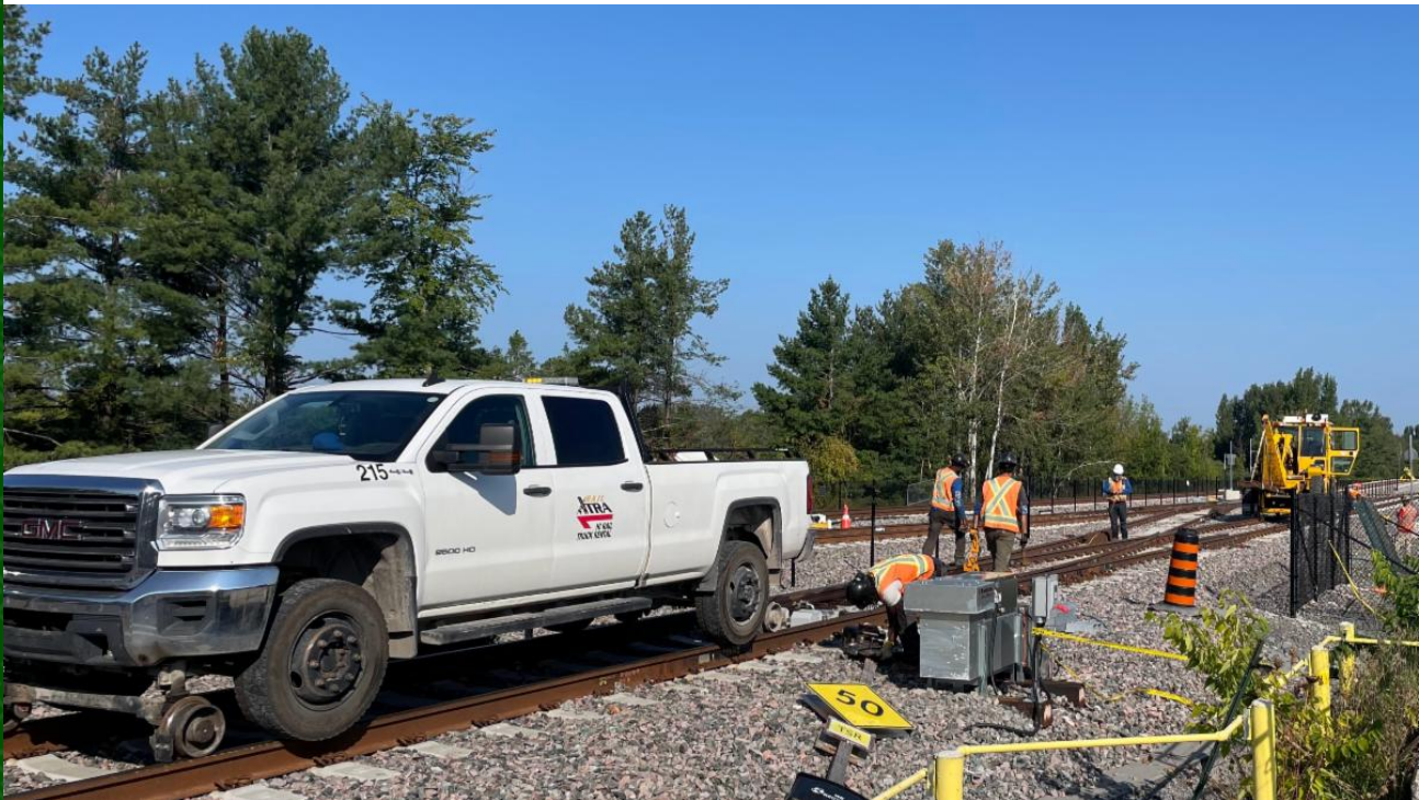
Ottawa Trillium Line - Crew working on switches at South Keys.
